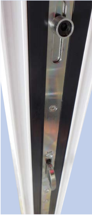
View of lower hook bolt and cam
