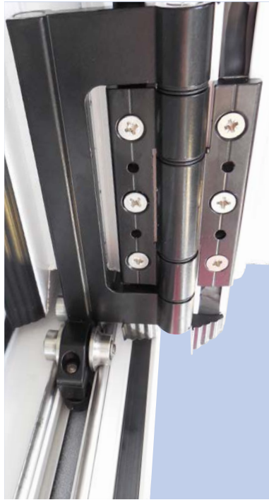
View of retained roller hinge
